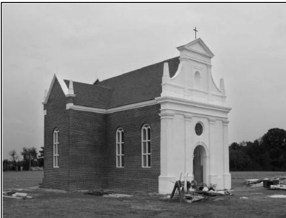
Figure 23. Reconstruction of the Brick Chapel.
